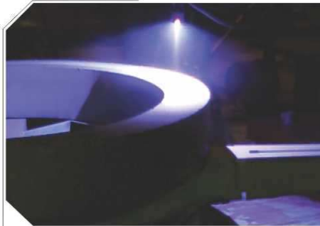
ANTI - CORROSION COATING ON WIND MILL PARTS
