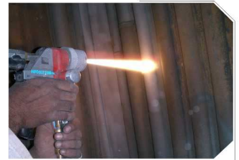
ANTI-EROSION & ANTI-CORROSION COATING ON BOILER TUBES
